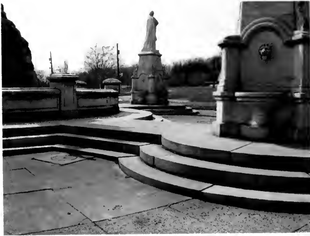
Figure 39: Granite stepped base (Photograph by author, March 2002)
